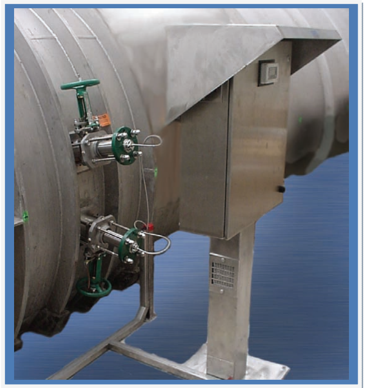
Split range, sealed metering System including an in-place calibration feature.
