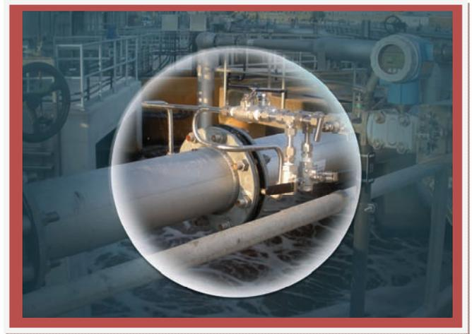
**Note the thickness of the Meter Center Flange is the only part of the meter that adds to the overall pipe length.**
